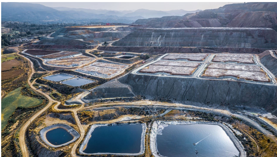
High-suction pressures are required to pull water from settling ponds on the surface.
