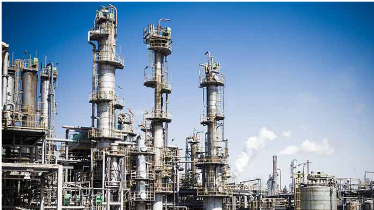
Image 4. Some environments dosing sodium hypochlorite (refineries or petrochemical plants) require API pumps.
